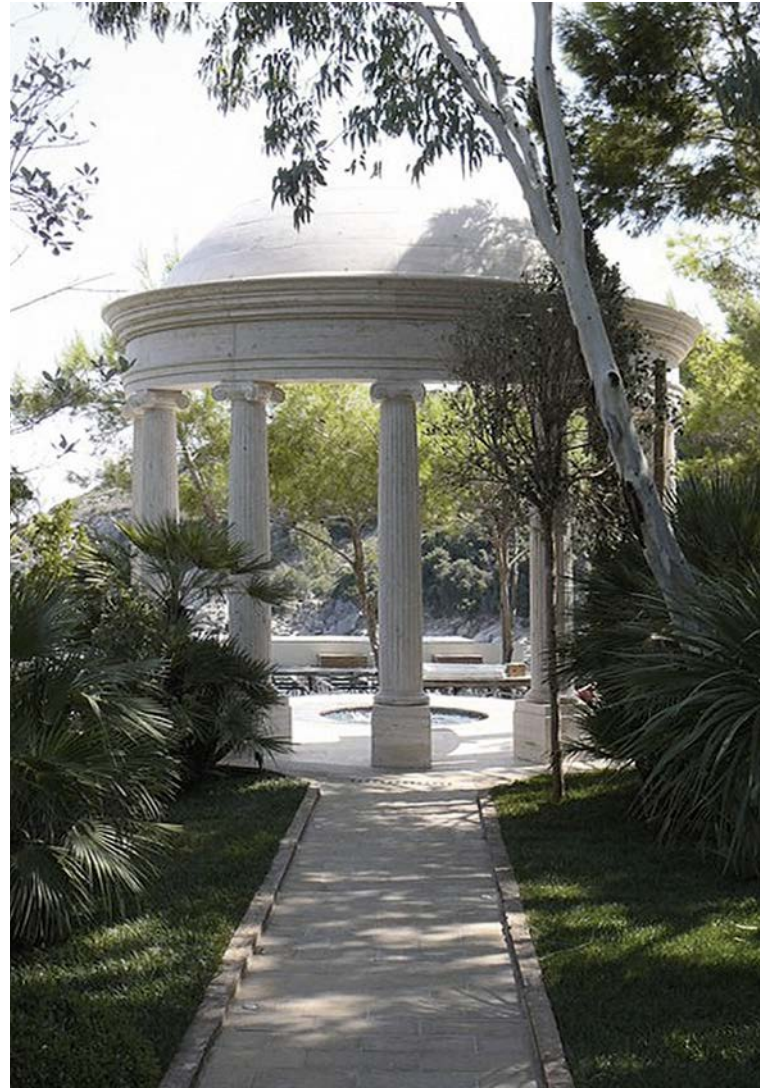
Rotonda in travertino con colonne ioniche e cupola monolitica. Travertine rotunda with Ionic columns and monolithic dome.
